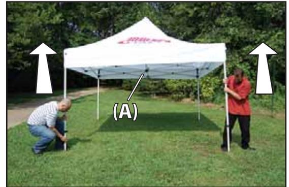
**Step 4:** With two people on opposite sides of the canopy frame, grasp the upper frame leg. While slightly lifting, pull in an outward direction, until frame is opened to full capacity. NOTE: the frame should NOT appear "tight" at this point.
